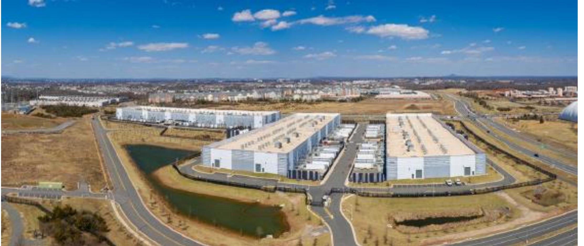
Data Center in Loudoun County Photo Credit: Hugh Kenny, Piedmont Environmental Council
